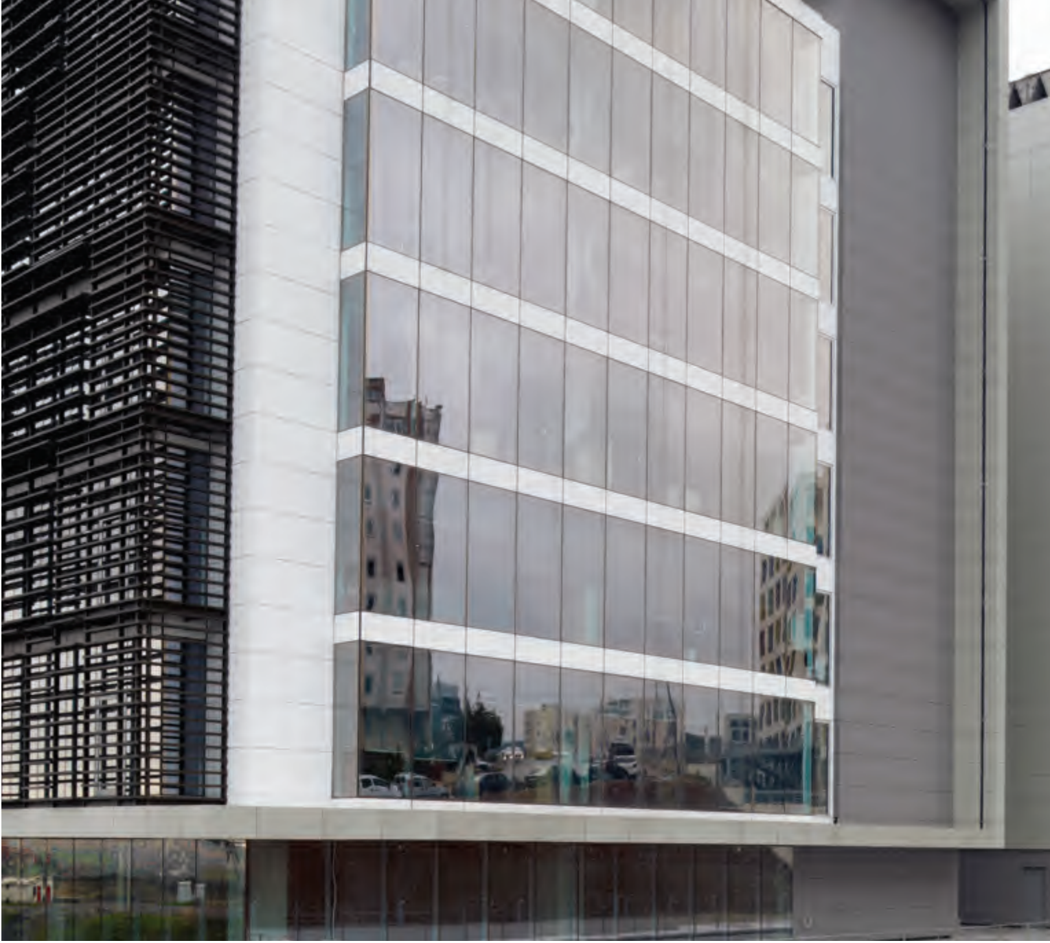
Kavacık İş Merkezi / İstanbul — Gizli Klipsli Sistem Kavacık Business Center / İstanbul — Hidden Clips Fitted Facade System
