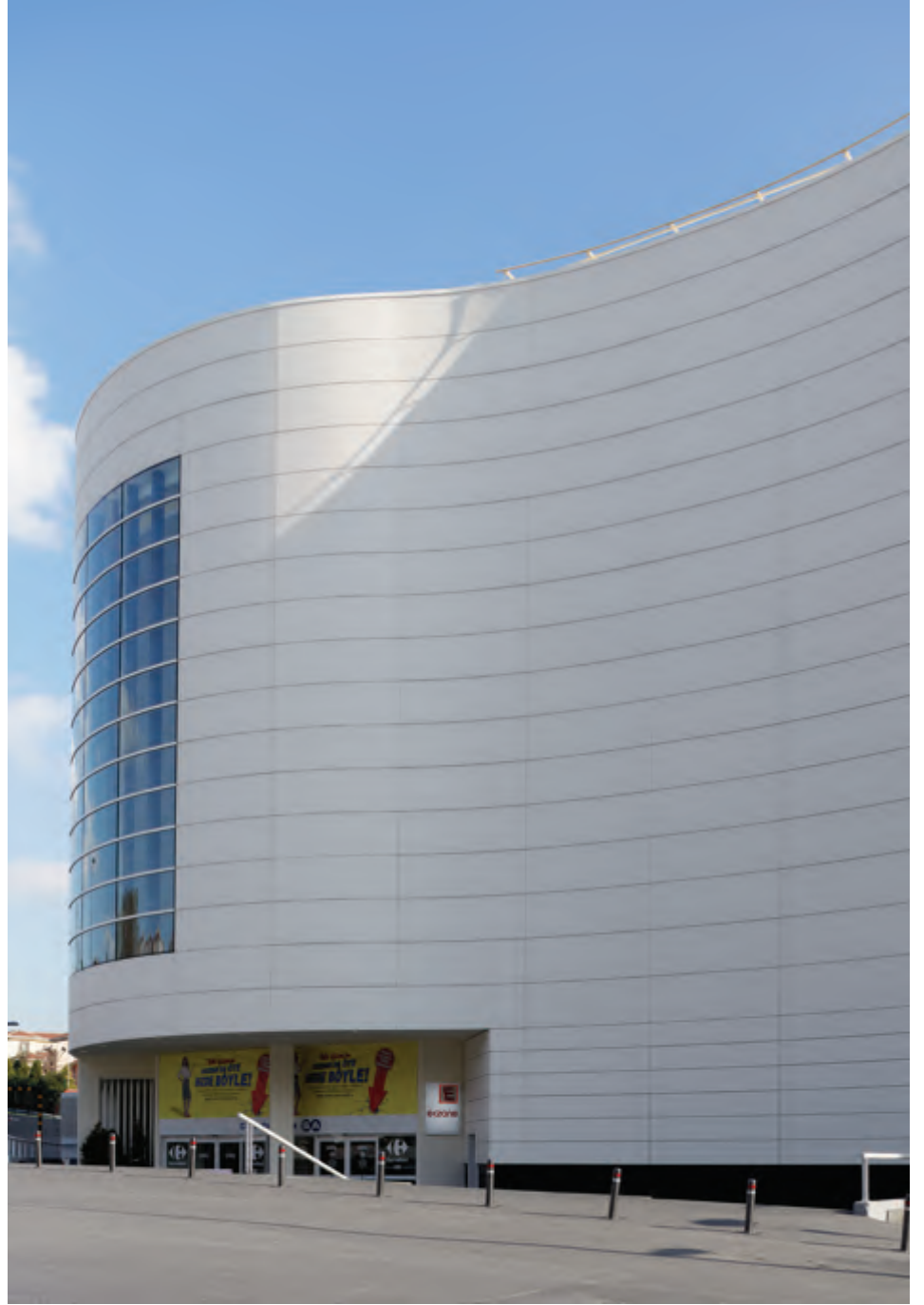
Carrefour AVM, Bahçelievler / İstanbul — Gizli Klipsli Sistem Carrefour Shopping Mall, Bahçelievler / İstanbul — Hidden Clips Fitted Facade System
